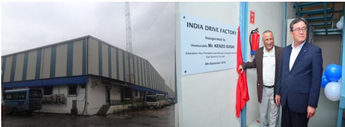
Fuji Electric India Drive Factory
